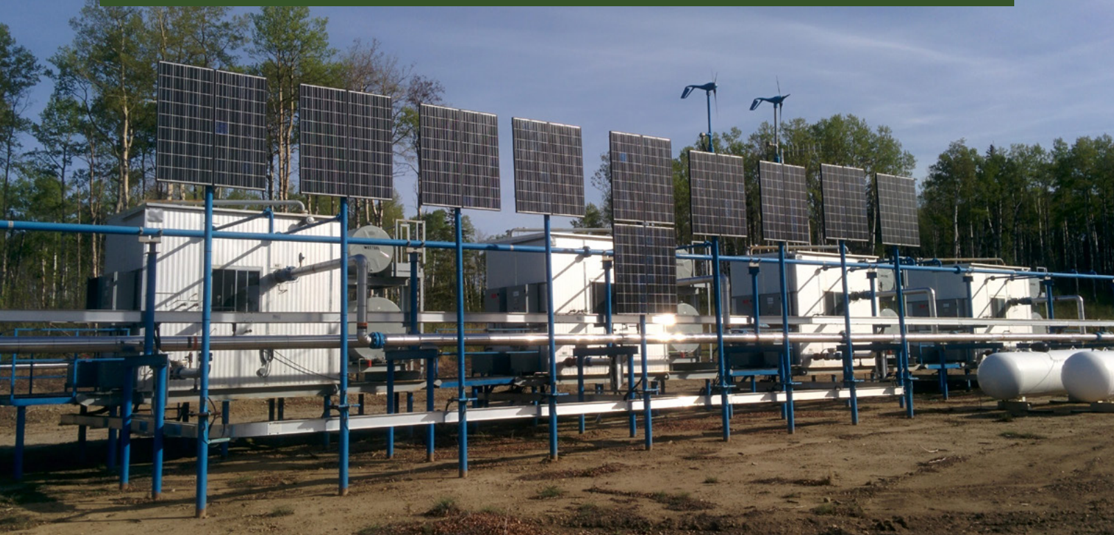
12-28-077-13W6M multi-well pad site with zero vented emissions and solar and wind electrified power generation
